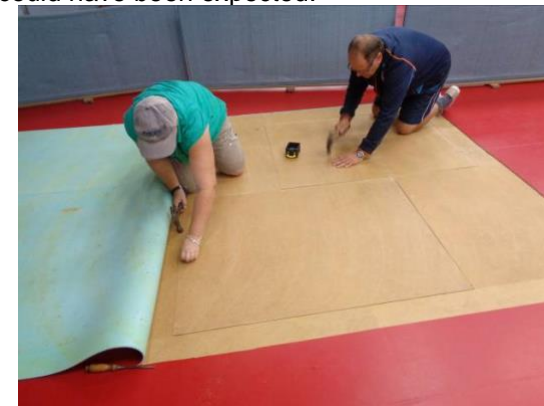
Cathy & Reinhard nailing the trimmed boards back onto the original floor before gluing and repositioning the Taraflex
